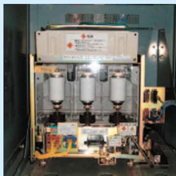
Renewed contactor manufactured in 2012 HN46AX-2S-HC vacuum magnetic contactor
